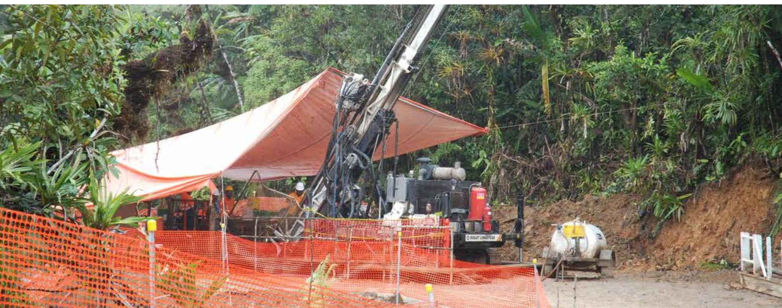
Drilling for core samples
