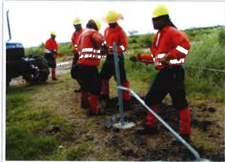
Site clearing and fencing
