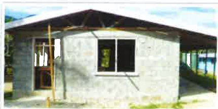
Namosi Primary School - new dining hall
