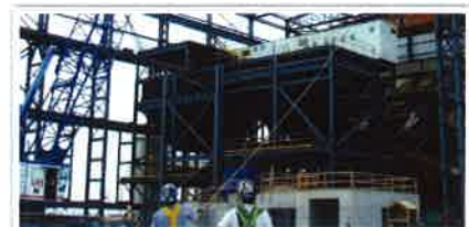
Constructing mine infrastructure
