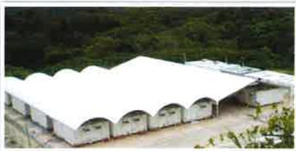
Camp, Offices and other facilities
