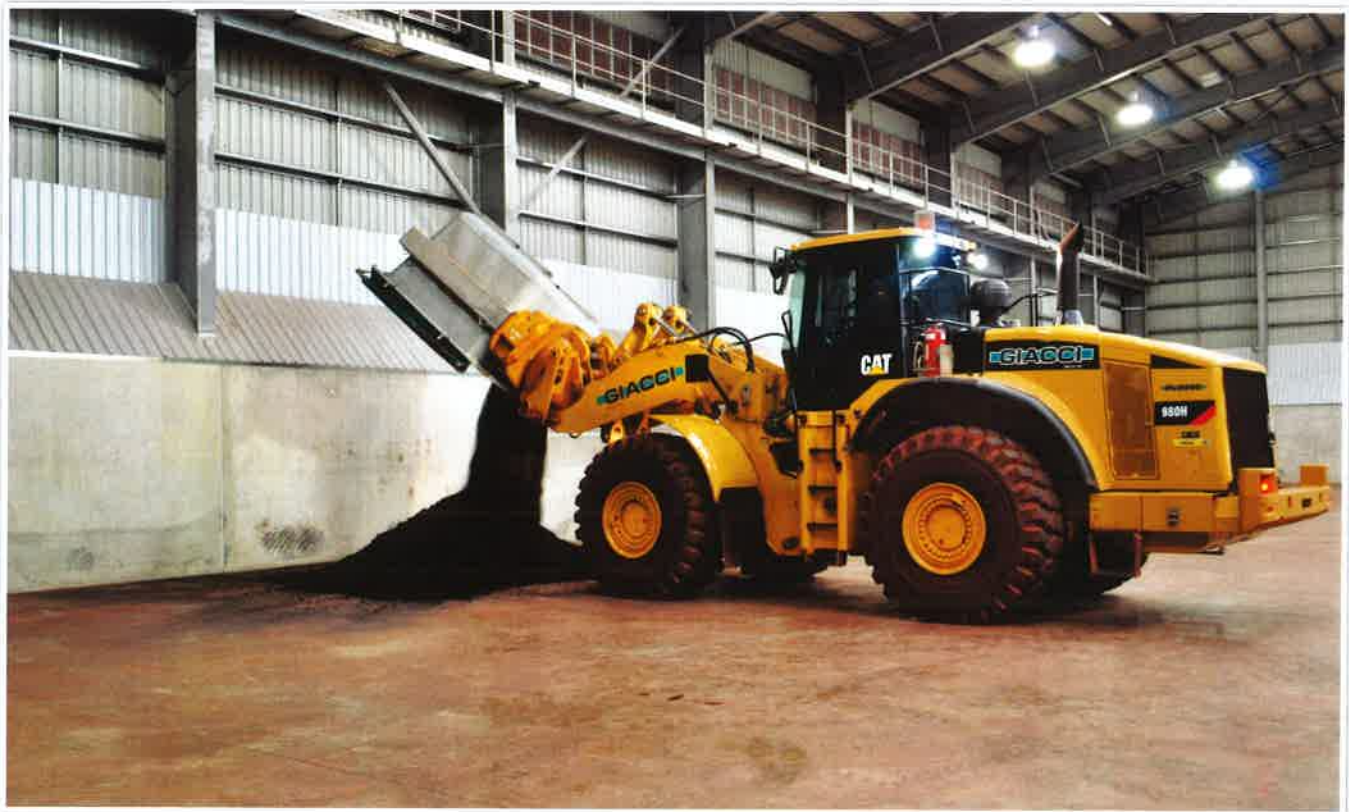
Enclosed concentrate stockpile building
